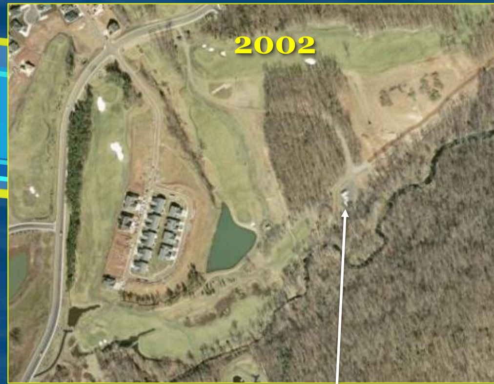
Sewage Pumping Station
