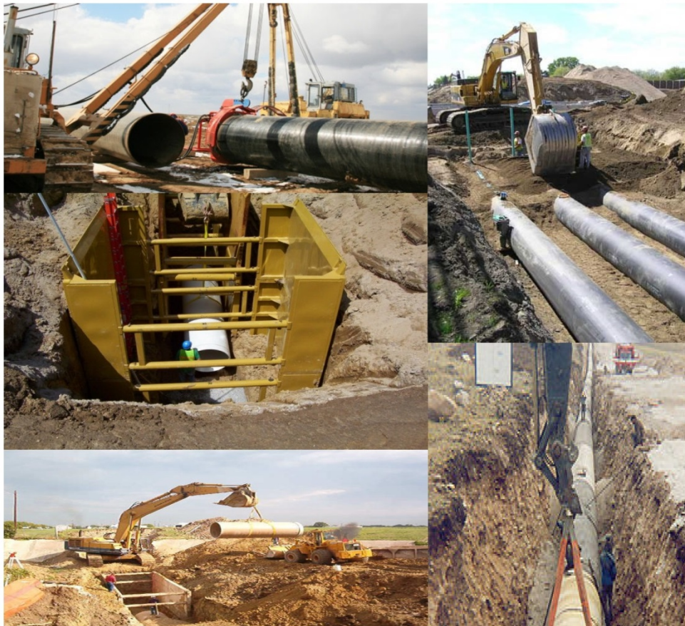
Water Transmission Projects
