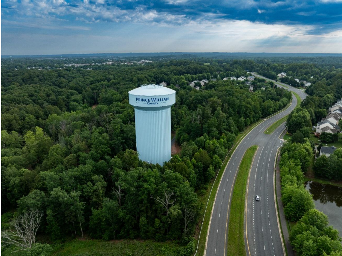
Prince William Water's elevated water storage tank along Prince William Parkway in Manassas.
