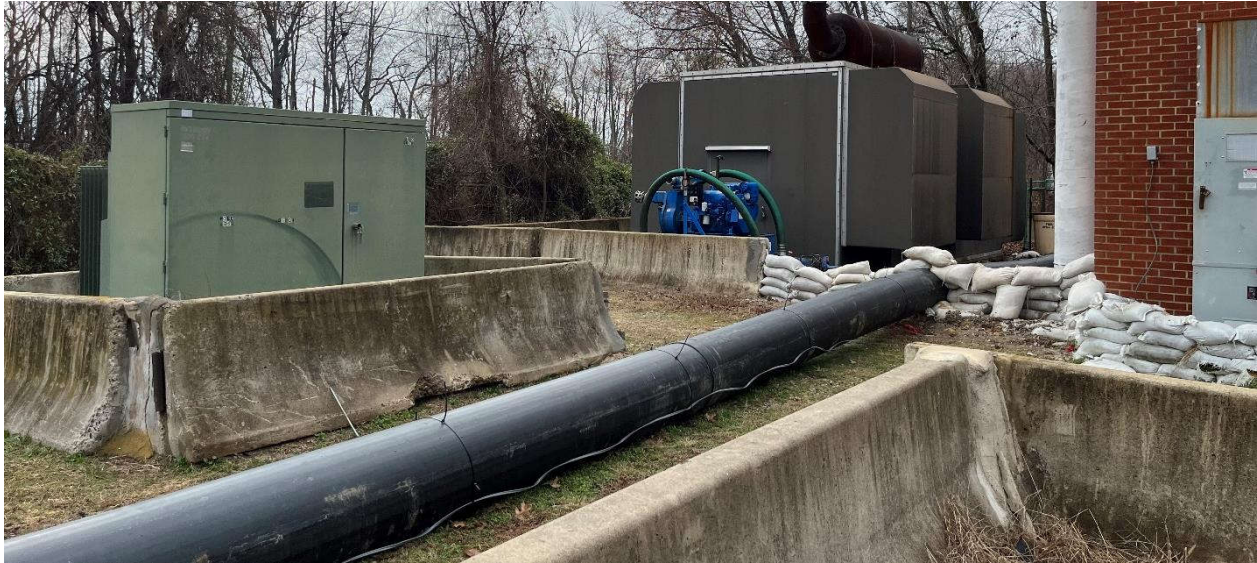
Figure 2.1 Pump Station Flood Protection
