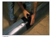
STEP 1 Wrap two or three layers of tape completely around the pipe where the tapping machine will be placed.
